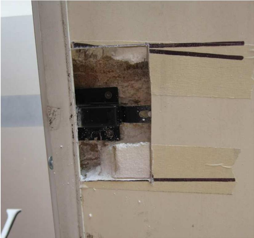
3. Using a 1/4 inch socket set with u-joint and 5/16 socket hold the nuts inside the panel so that you can unscrew them with a Philips head screw driver from the outside. Don't lose the nuts, you will need them in reassembly.
