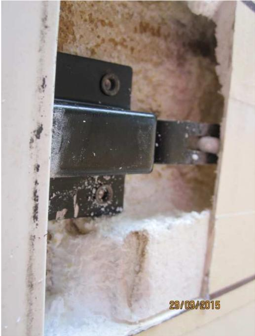
4. With the latch rod disconnected (in the door middle) you can now slide the latch towards the center until you can tip it out of the hole in the door with the wide edge of the latch first.
