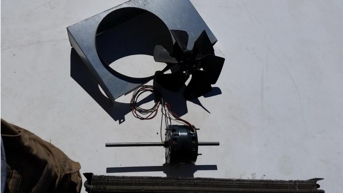
Installation is the reverse of the removal. Once you have the sheet metal panel mounted on the back of the new motor using the same nuts you took off, install the fans and tighten up the clamps. Now reinsert the motor and reinstall all the sheet metal using the screws you took out. ( I put all the screws in the AC pan so they wouldn't roll off the roof)
