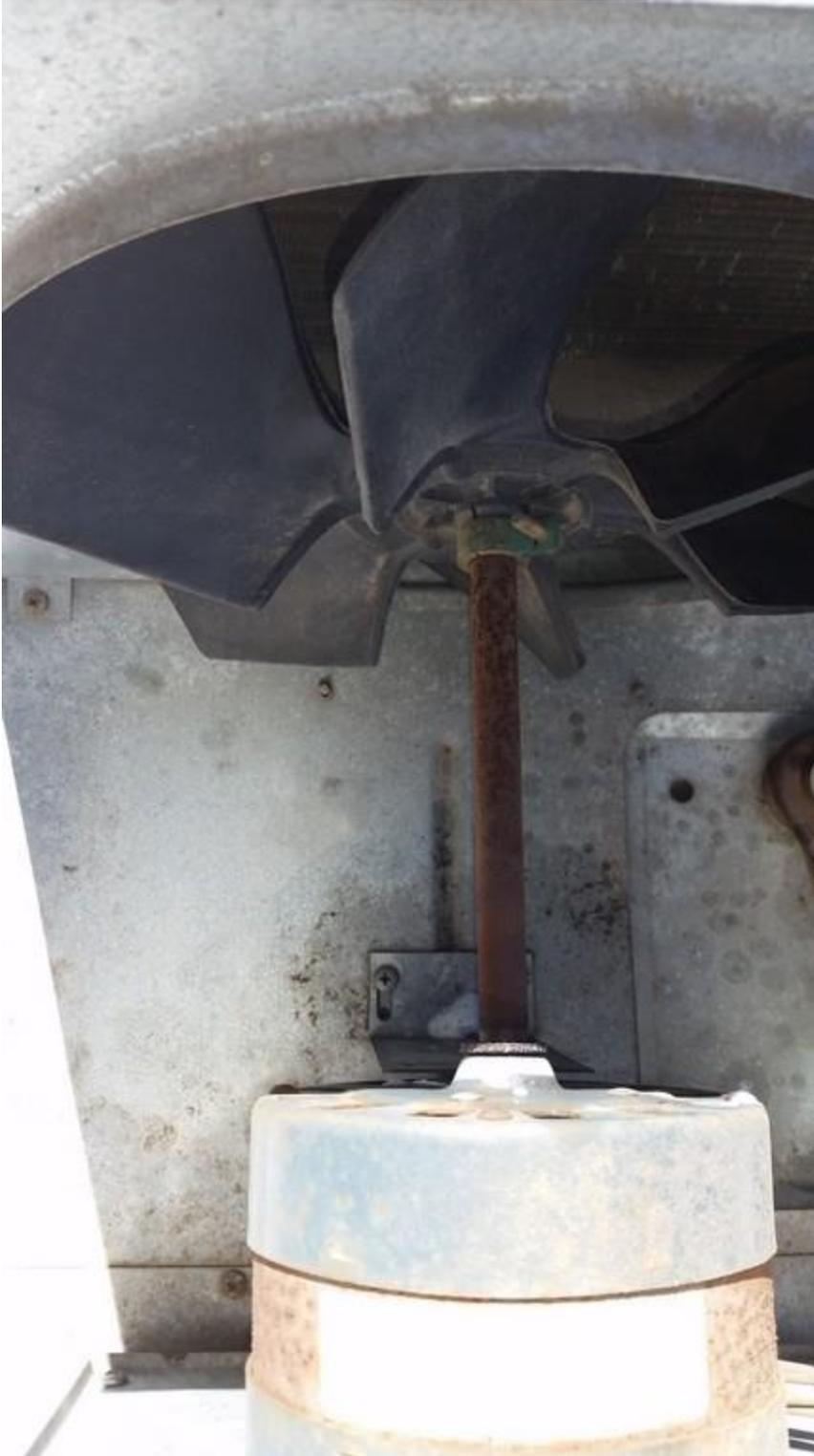
There are two fans, the bladed fan you see at the top of the above photo and a squirrel cage fan hidden in the sheet metal. Using the 5/32 Allen wrench, remove the clamp that holds the fan blade on. Squirt some penetrating oil on the shaft. It's no doubt rusty. Remove the sheet metal screws that hold the sheet metal surround of the coil and fan. Then remove the 4-5 screws that hold the panel that the rear shaft goes
